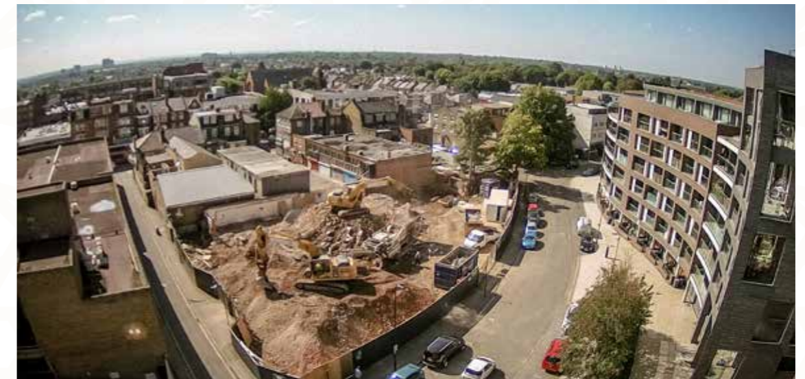
WLIC Construction Site September 2017
