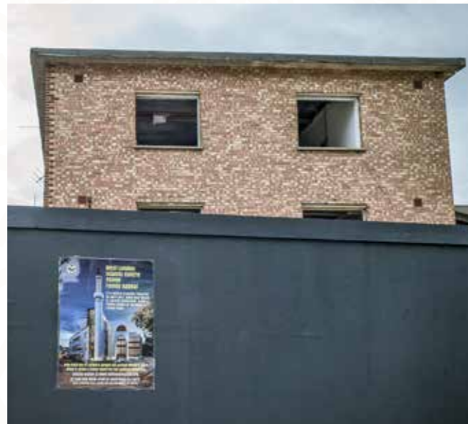
Preparations for WLIC Demolition
