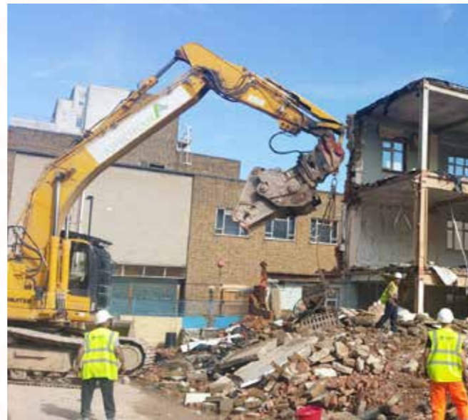
WLIC Demolition Works Begin August 2017
